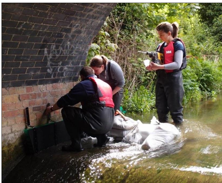
Figure16: A 'bristle board' eel pass being installed on the River Darent with the North West Kent Countryside Partnership.
