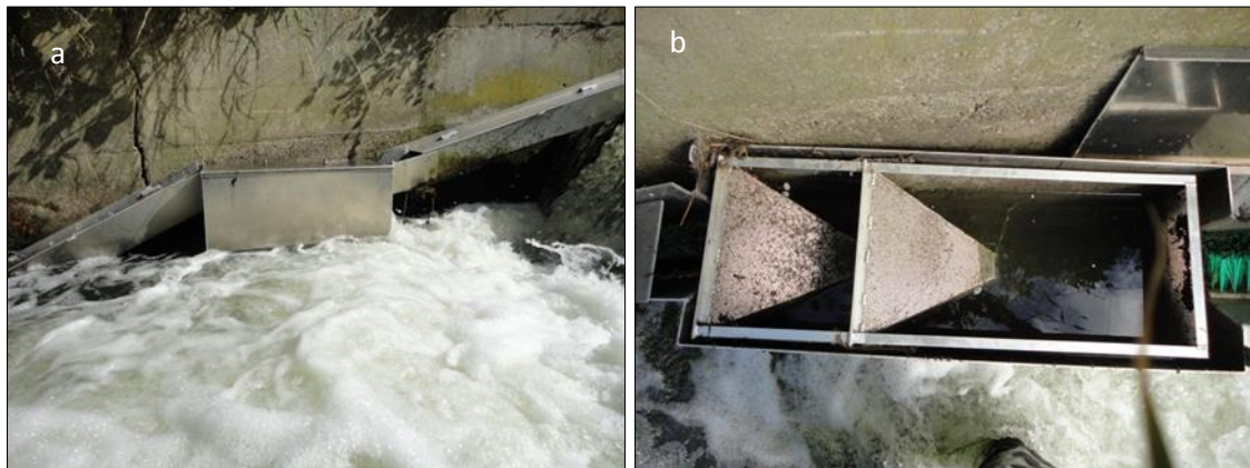
Figure 10: a, The eel pass with trap on the Hogsmill River at Middle Mill and, b, open lid aerial view of trap .
