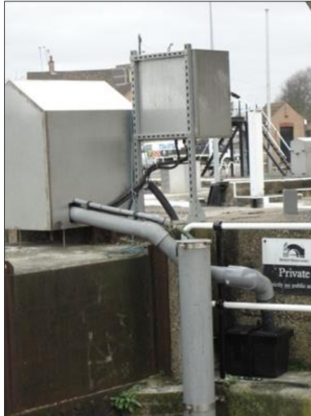
Figure 12: The modified eel pass with trap at Bow Locks on the River Lea
