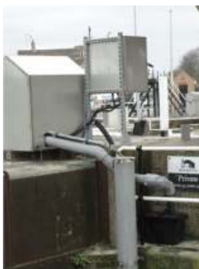
Figure 10: The modified eel pass with trap at Bow Locks on the River Lee
