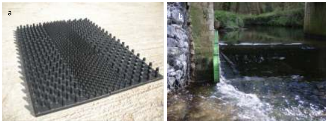
Figure 13: a) an eel pass tile and, b) a simple bristle board pass
