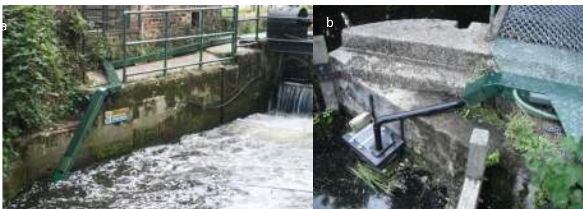
Figure 11: a) the eel pass and, b) trap at Merton Abbey Mills on the River Wandle.
