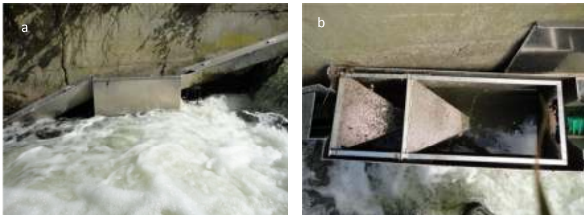
Figure 12: a) The eel pass with trap on the Hogsmill River at Middle Mill and, b) open lid aerial view of trap .
