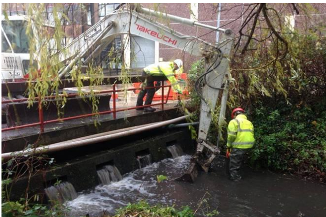
The weir at the Coors brewery about to be removed
