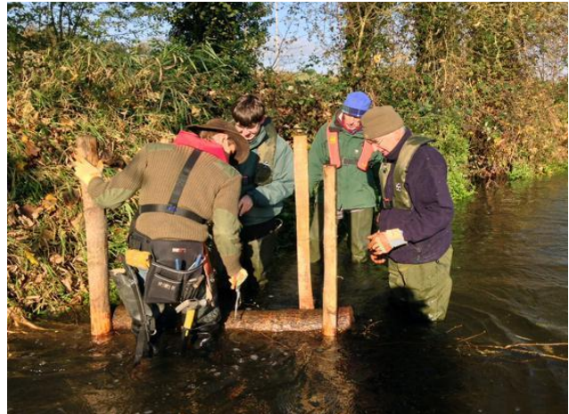
Fisheries Officer Matt Drew, with the help of volunteers, fixes a large woody debris flow deflector into the Wye.
