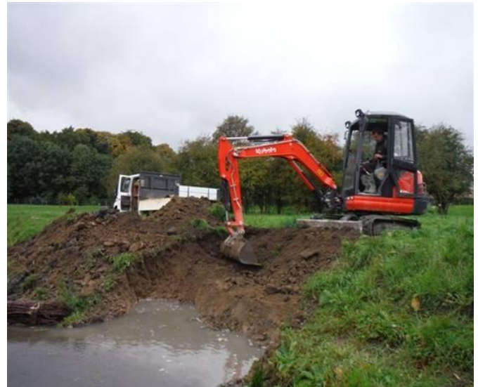
Work starts on the creation of the first of two cattle drinks on the Wey at Wrecclesham
