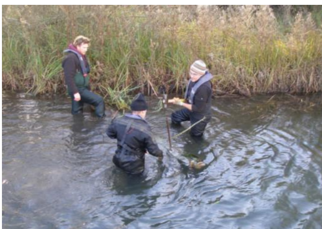
A flow deflector gets firmly fixed in place to the river bed
