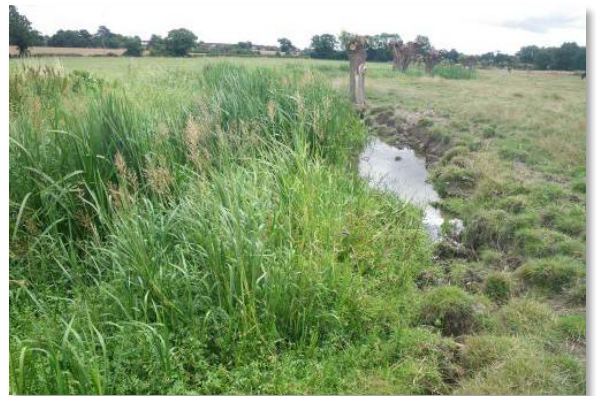
Before: a reed-choked channel with poor flow
