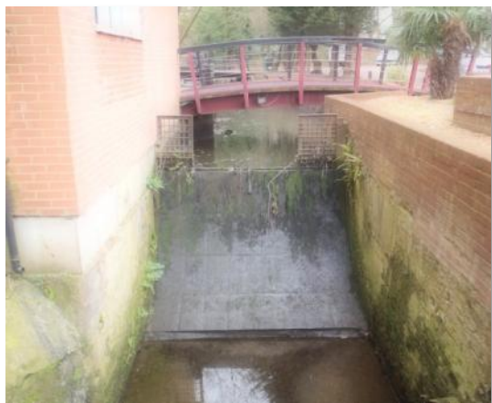
Pledges Mill weir three metres high a total barrier to fish passage
