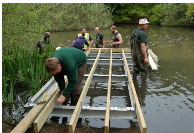
Volunteers constructing the new angling platforms in Epping Forest.
