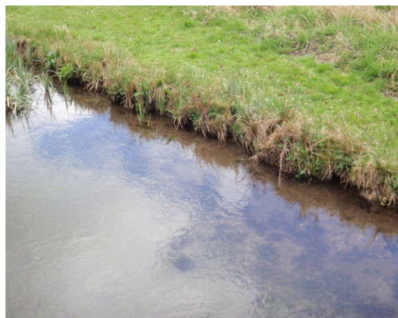
Heavily managed bank. Provides no cover, very little habitat, no protection from erosion and is visually unattractive.
